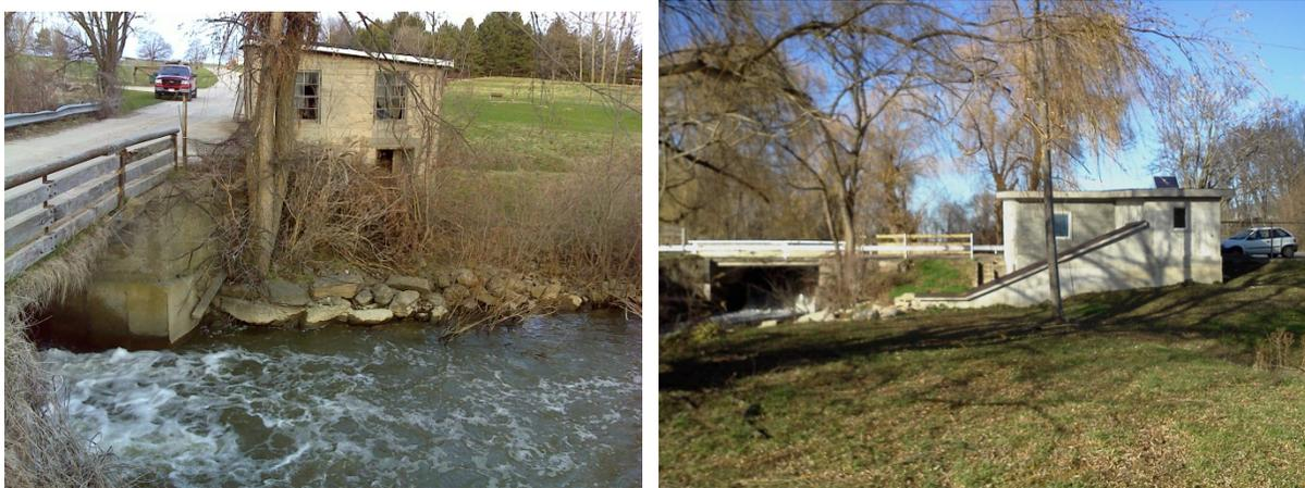
**Figure 2. Site of Fletcher's ASG installation before work began on the site (left) and after installation was complete (right). The access road is located on the dam crest, and the pre-existing dam spillway is visible under the roadway on the left side of both images.**
